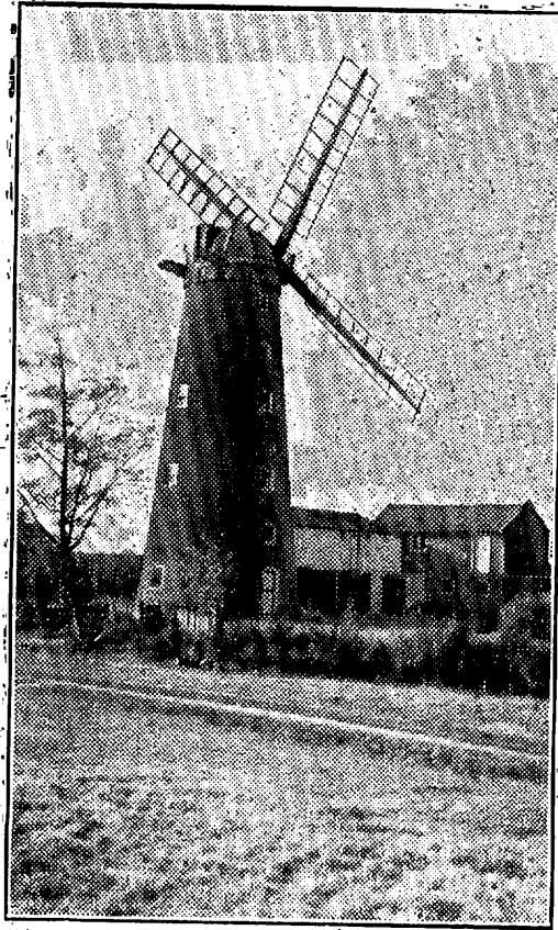
TO BE PRESERVED. —Buttrams tower mill, Woodbridge, Suffolk, one of the windmills selected in a recent report by the East Suffolk County Council as most suitable for preservation.
